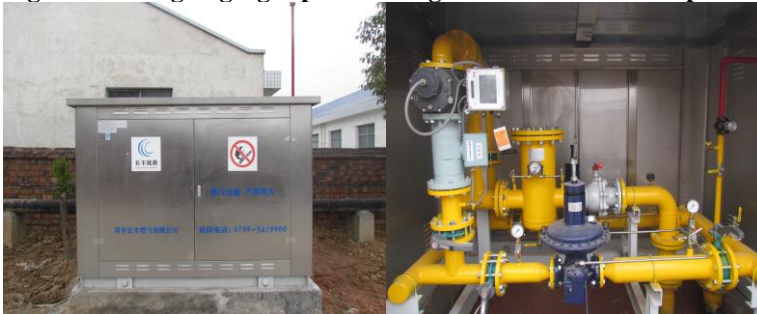
Figure 1: Changfeng's gas pressure regulator in the ceramic plant
